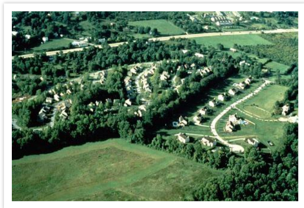
The two adjacent developments pictured above illustrate conservation design (left) versus traditional design (right)
