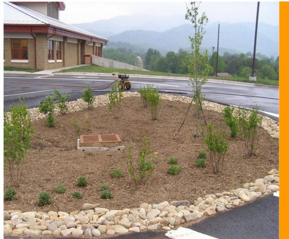
Raingardens and other BMPs collect runoff from parking lots at Bethel Elementary School
