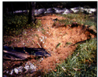
To reduce stream sedimentation, silt fences must be properly installed and then maintained.
